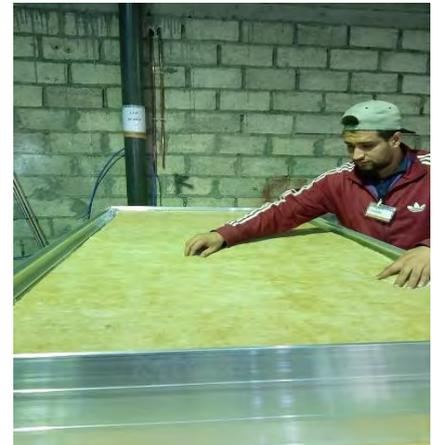
Figure 107 Insulation placement inside the frame casing [3]
