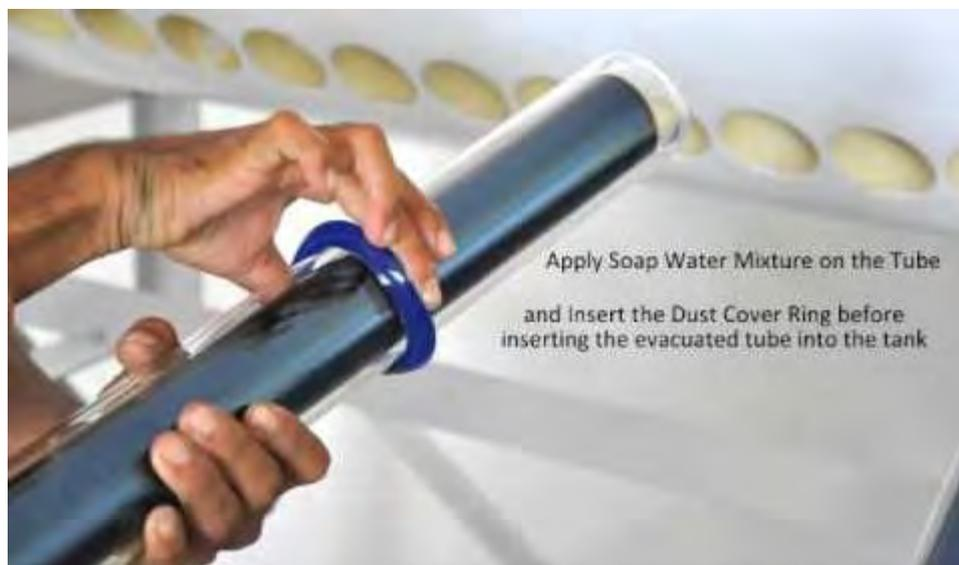
Figure 118 Assembly of evacuated tube with storage tank
